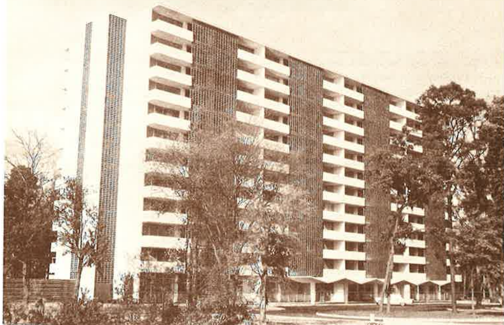
View of the beautiful Riverton Tower, home of the Jacksonville Division, just prior to occupancy in September 1963.
